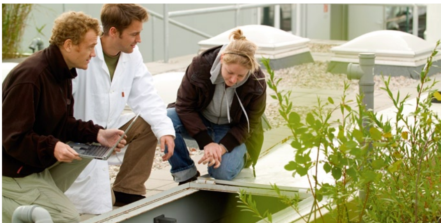
In the pilot plant of the project "Compartment Transfer" (CoTra) various semi-natural remediation techniques are being tested to eliminate BTEX aromatic compounds in the groundwater.
