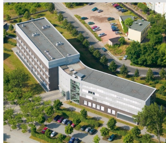
UFZ offices in Magdeburg, Brueckstrasse 3a
